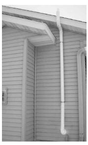
**Figure 9** Vent Line Installation (3 inch)
