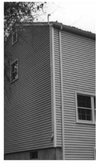
**Figure 8**Vent Line Installation (2 inch)
