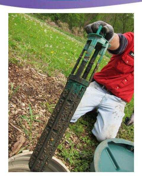
Effluent filters shown visually loaded
